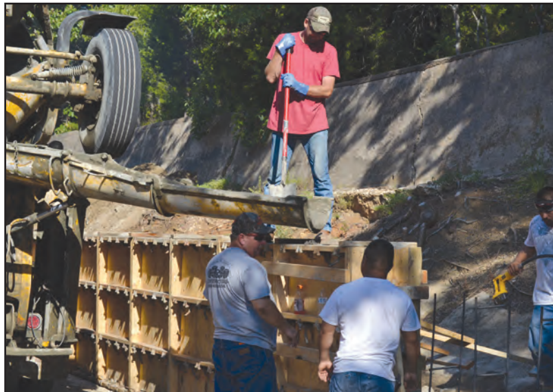
A new concrete wall behind the Bill H. Hill Library on Eastern's Wilburton campus kicked off a series of campus improvements now in the works. Photo by Jamie Fink
